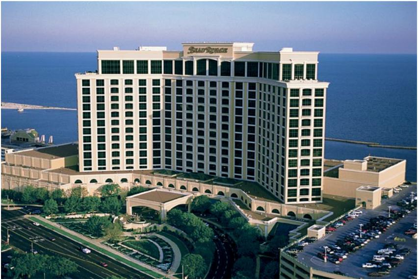
**Figure 2-2** The guest rooms of the Beau Rivage Casino in Biloxi, Mississippi, are raised above a massive base, built after Hurricane Katrina damaged the building in 2005. The base serves as a bulwark against storm surge and is built to accept some flooding. Massive structures along a coastline can deflect storm surges on to other properties, so they should be constructed as part of a coordinated storm protection strategy.
