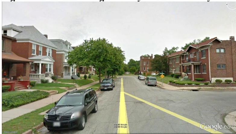
Figure 2-3B: Mix of Single Family and Multifamily Buildings in Compton Heights
