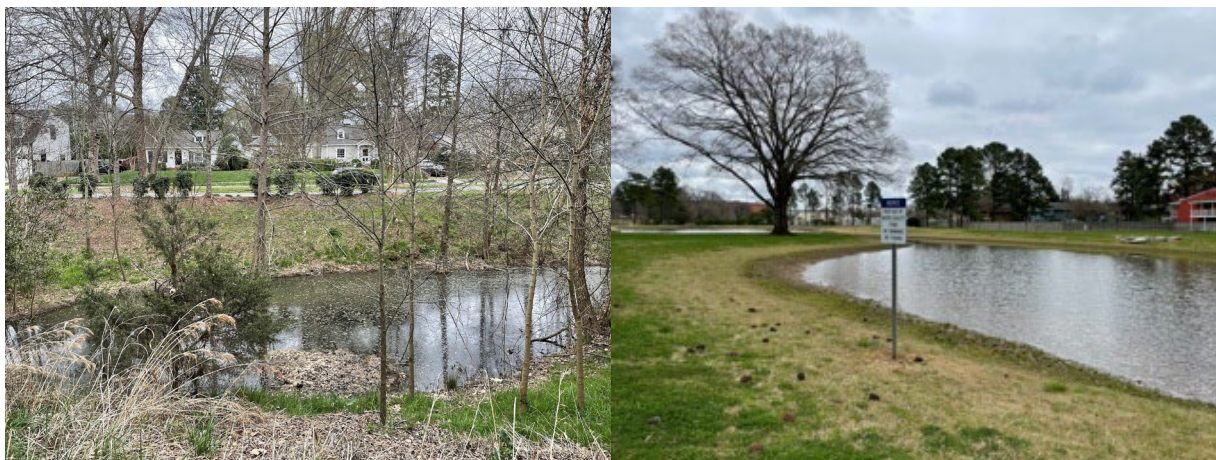
Figure 1. A water filtration retention system (left) and detention basin (right) constructed on bought out properties in Charlotte Mecklenburg County, North Carolina.
