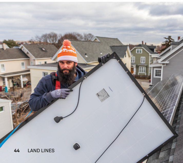
A solar installer in Lowell, Massachusetts. Credit: Jerry Monkman/ EcoPhotography.
