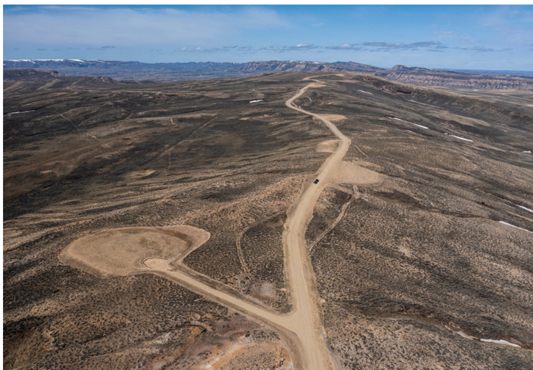
Pads have been cleared for wind turbines at Wyoming’s Overland Trail Ranch, which straddles the Continental Divide. Credit: Robert Gauthier/ Los Angeles Times.
