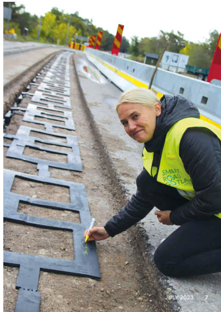
Embedding wireless charging coils in a road in Gotland, Sweden, for a demonstration project led by Electreon. Credit: Electreon.
