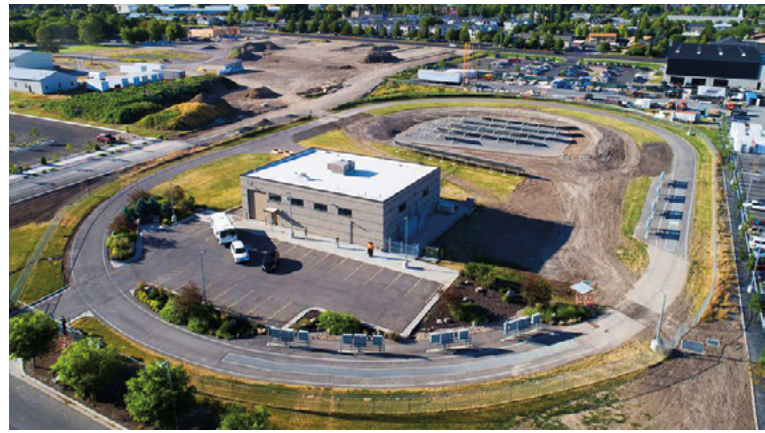
The ASPIRE Engineering Research Center test track in North Logan, Utah, site of a roadway electrification demonstration project that uses wireless charging technology provided by Electreon. Credit: Courtesy of ASPIRE.
