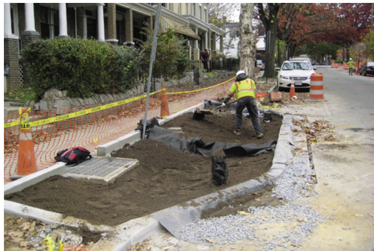
Installation of a bioretention bumpout in Washington, DC, where a Green Bonds program provides capital for stormwater and sewage management projects. Credit: Chesapeake Stormwater Network.
