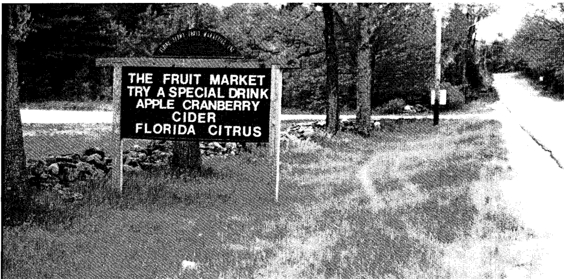
Free-standing sign (with changeable message) suitable for commercial roadside. Constructed with 6" x 6" posts and beams (pressure-treated), and exterior grade plywood mounted with indoor-outdoor carpeting. Lightweight plastic letters are held in place by postage stamp-sized "Velcro" tabs.
