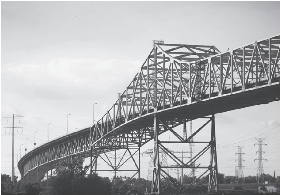
Figure 7.2 Main Span of the Chicago Skyway
