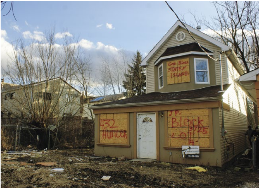
Hurricane Sandy caused major damage to homes and infrastructure on Staten Island, as seen in January, three months after the storm. Photo by Laurie Johnson (2013).
