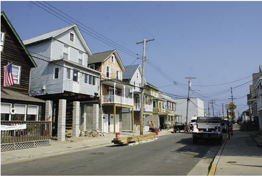
In October 2013, housing repairs involving floor elevations to mitigate future flood risks were under way in the Borough of Sea Bright, New Jersey. Photo by Laurie Johnson (2013).
