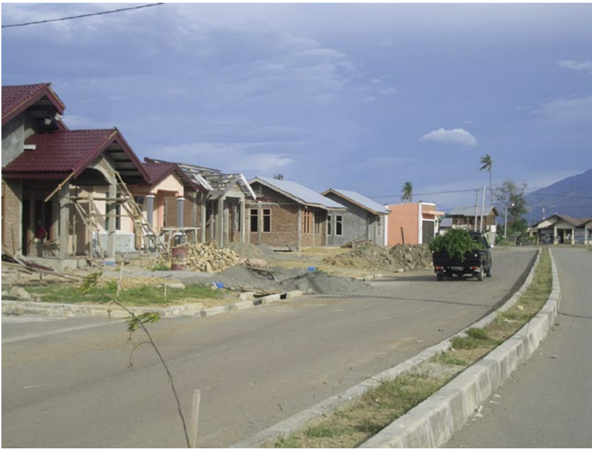
Most of the damaged housing in Banda Aceh was reconstructed within five years of the tsunami. Photo by Robert Olshansky (2008).
