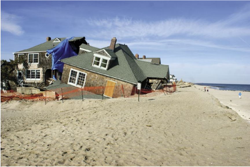
Hurricane Sandy damaged many homes along the New Jersey shore after making landfall there on October 29, 2012. Photo by Laurie Johnson (2013).
