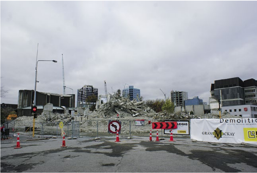
The central business district of Christchurch was cordoned off for more than a year to help ensure public safety from aftershocks and facilitate the demolition of damaged buildings. Photo by Laurie Johnson (2012).
