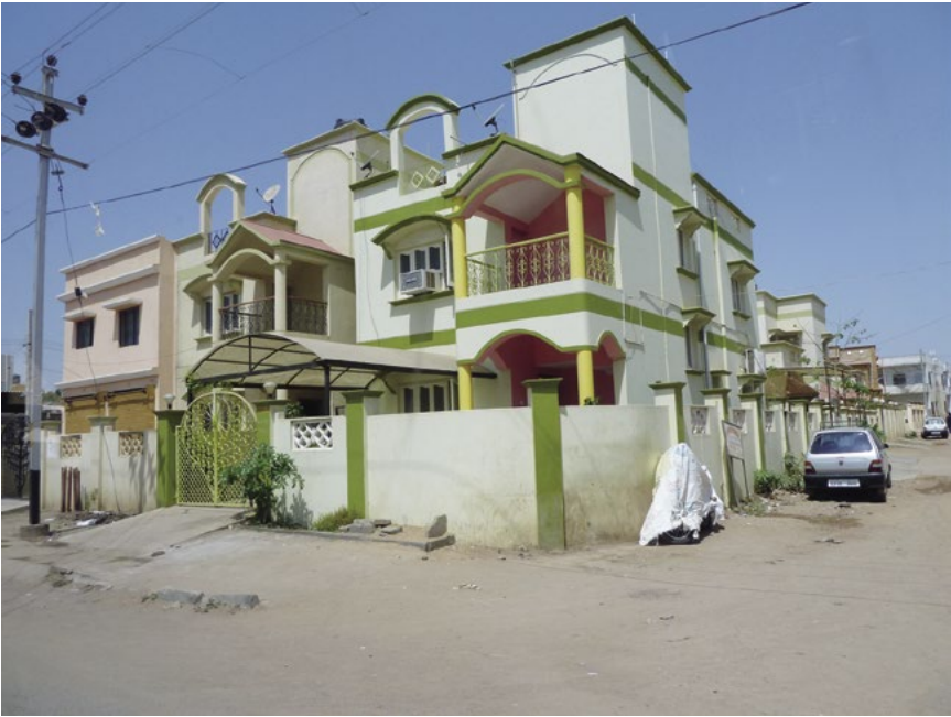
Approximately 200,000 housing units, such as these in Bhuj, were reconstructed after the 2001 earthquake in India. Photo by Robert Olshansky (2011).
