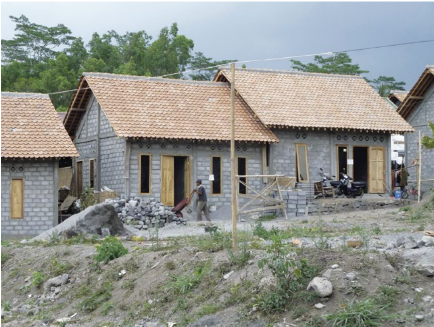
New housing in dense villages was constructed for families relocated from the volcanic hazard zones. Photo by Robert Olshansky (2012).
