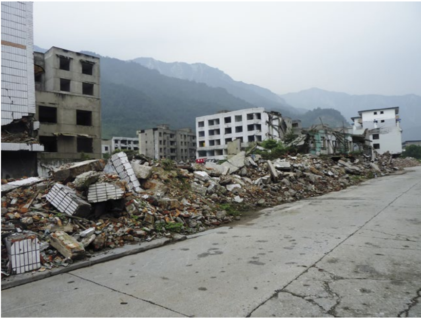
The 2008 earthquake caused severe damage to numerous cities throughout a wide region of China, including most of the industrial town of Hanwang, Mianzhu City. Photo by Robert Olshansky (2011).
