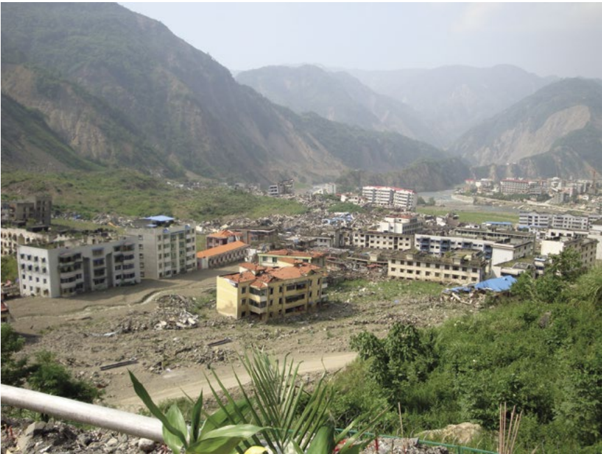
The city of Beichuan, shown in 2009, was seriously damaged and abandoned as a result of the 2008 earthquake. Photo by Robert Olshansky (2009).
