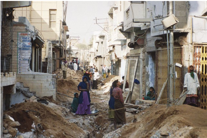
In 2004, a sewer line was laid in Saraf Bazaar in the heart of the old city of Bhuj as part of the land-readjustment process. Source: Photograph by B. R. Balachandran, Environmental Planning Collaborative, Ahmedabad, during the preparation and implementation of Town Planning Schemes for Bhuj in the period from 2001 to 2004. Reprinted with permission.
