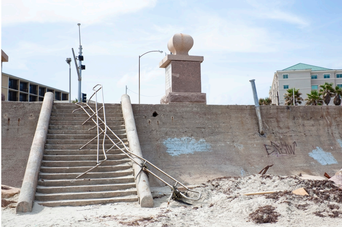
The sea wall on the East Coast of Galveston Island stands as a buffer between the mighty forces of the Gulf and the city of Galveston. Eight months after Hurricane Ike hit Galveston in September 2008, the sea wall and beach remained in the upheaved condition left by Ike. Source: fstop123/iStock/Getty Images Plus
