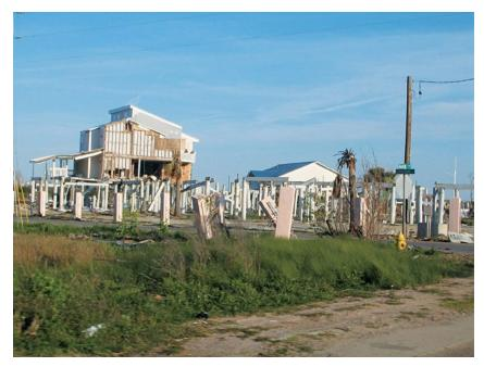
Figure 2-3 Raising buildings on structural columns will not protect against the velocity of a storm surge. This photo shows the forty-unit Spinnaker Point condominiums in Pascagoula, Mississippi, after flood tides and a storm surge from Hurricane Katrina in 2005. Raised houses along the New Jersey Shore suffered comparable damage from flood surges during Superstorm Sandy in 2012.
