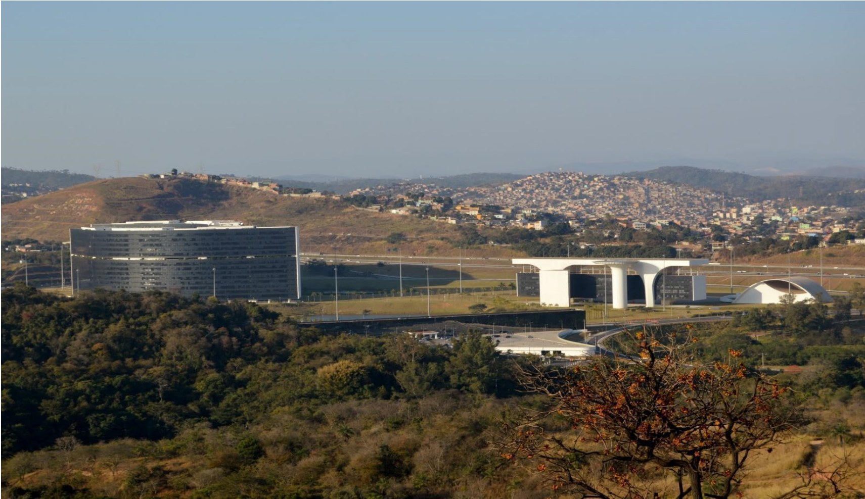
In the foreground, the Palácio Tiradentes (right) and the Edifício Gerais (left). In the background, the Green Line and part of the São Benedito District in Santa Luzia. Source: Clarissa Veloso (August 2017)
