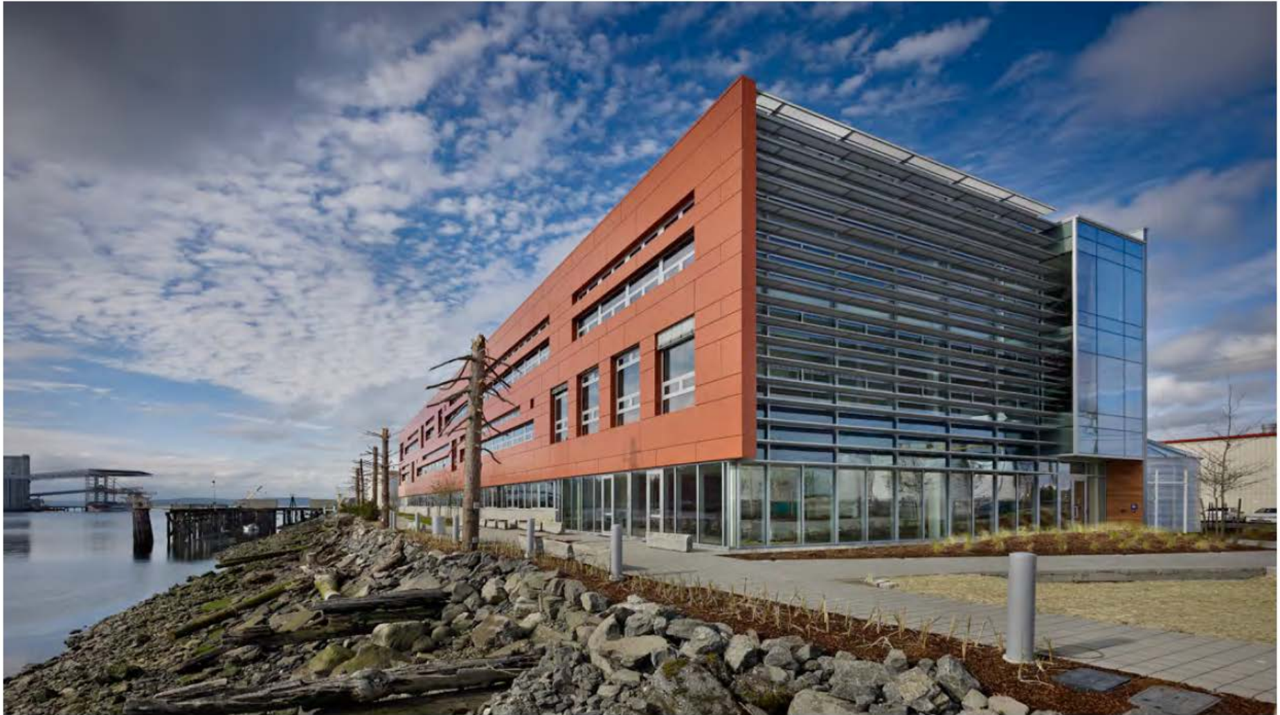
Center for Urban Waters An NDC Public-Private Partnership Project
