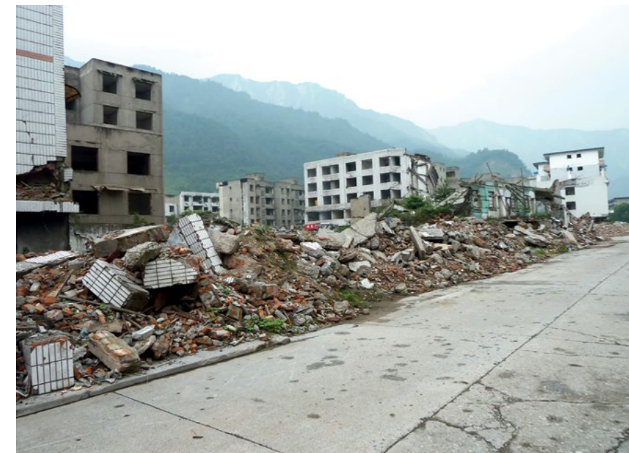
The 2008 earthquake in the Sichuan province of China caused severe damage to numerous cities throughout a wide region, including most of the industrial town of Hanwang, Mianzhu City. Credit: R. Olshansky (2011).
