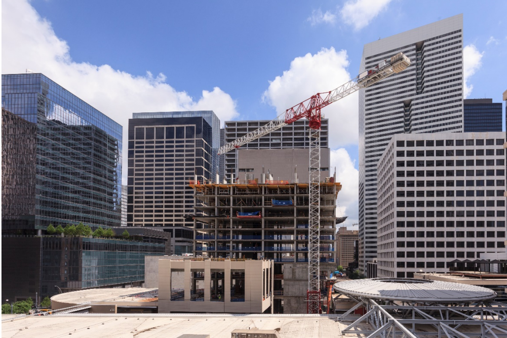
Photo: Construction site in Houston downtown district. Credit: Getty Images/typhoonski.
